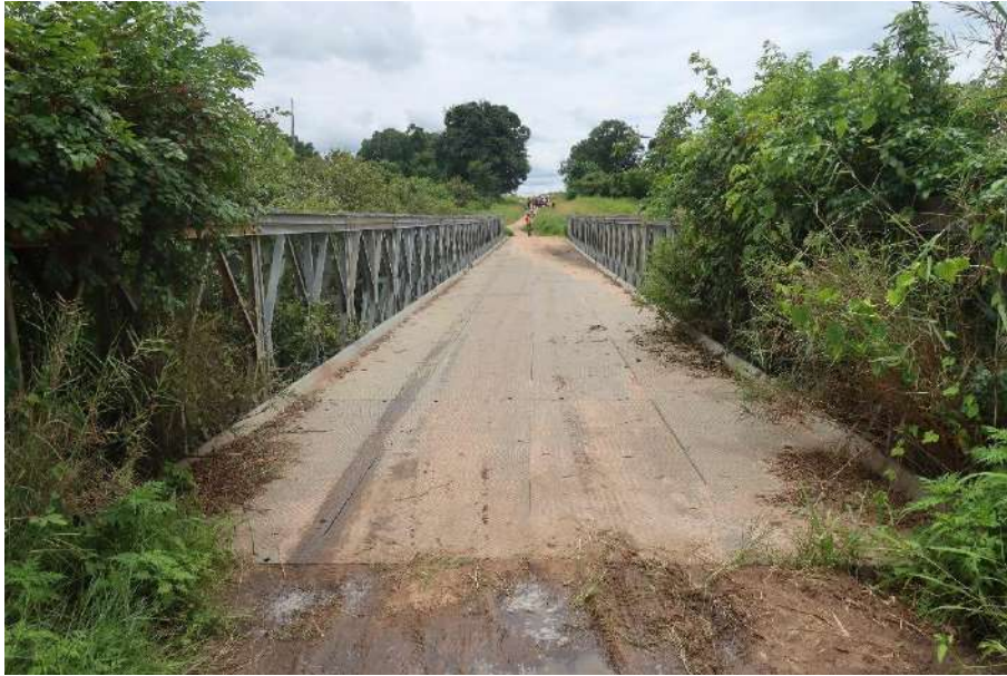
Figure 14 – Photographic record of the bridge located at PK 39+175.
