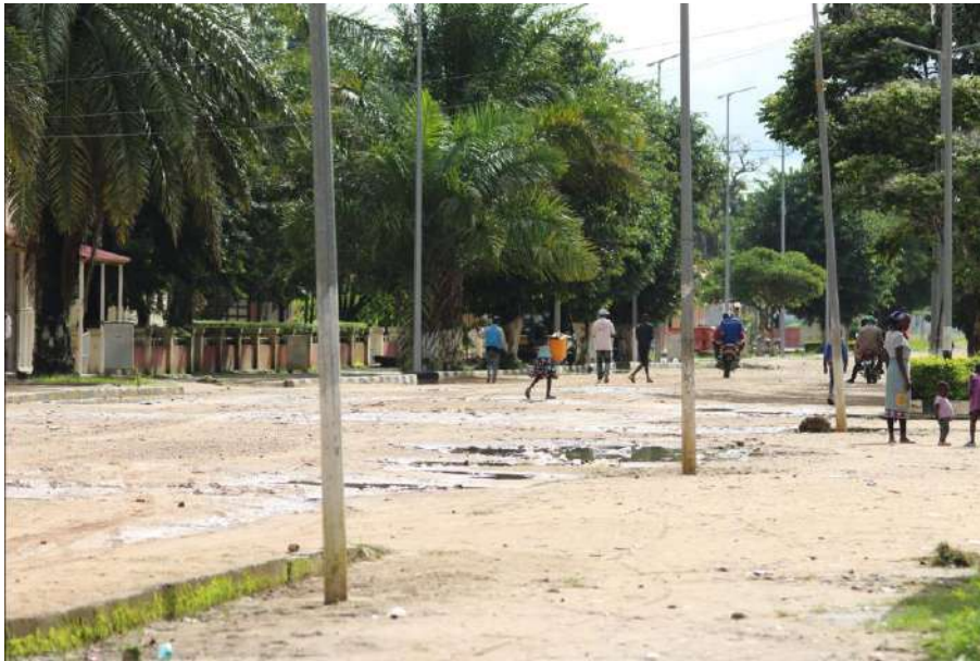
Figure 120 - Photographic record of domestic wastewater (sewage) flowing in the open.
