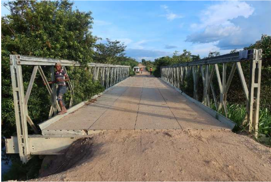
Figure 10 – Photographic record of the bridge located at PK 79+400.
