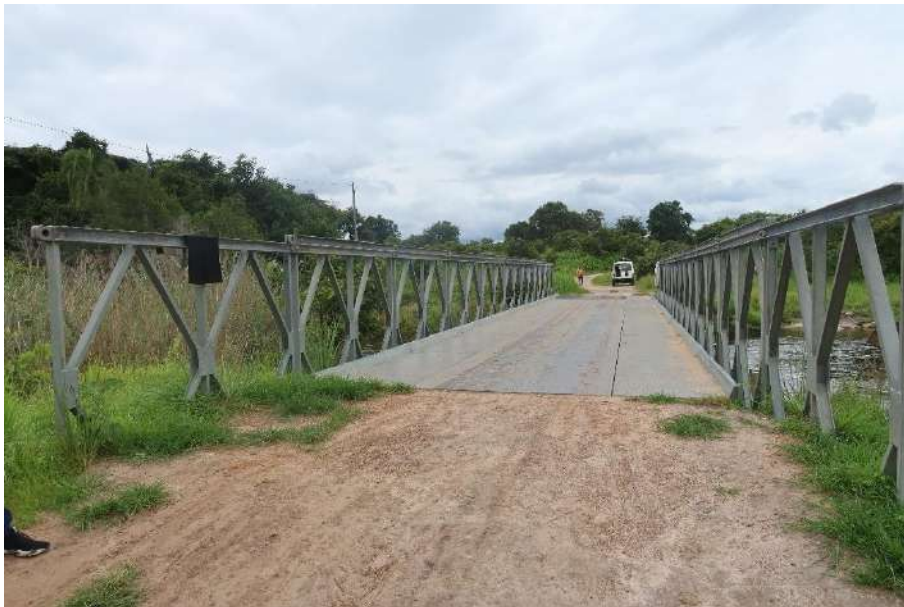
Figure 13 – Photographic record of the bridge located at PK 27+450.
