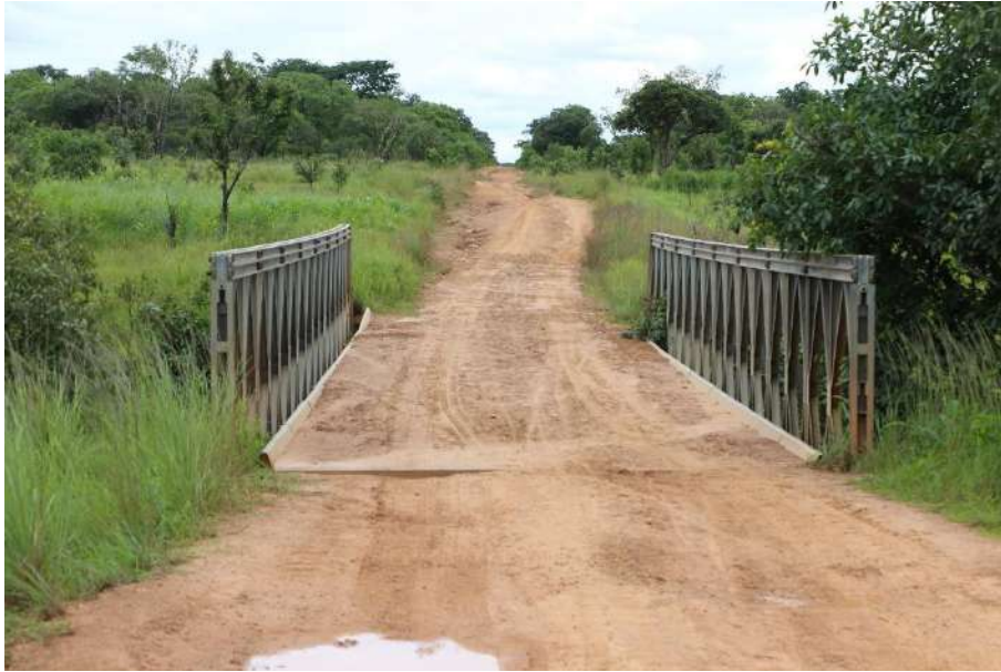
Figure 12 – Photographic record of the bridge located at PK 118+500.
