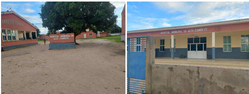
Figure 208 – Photographic record of the Municipal Hospital of Alto Zambeze.
