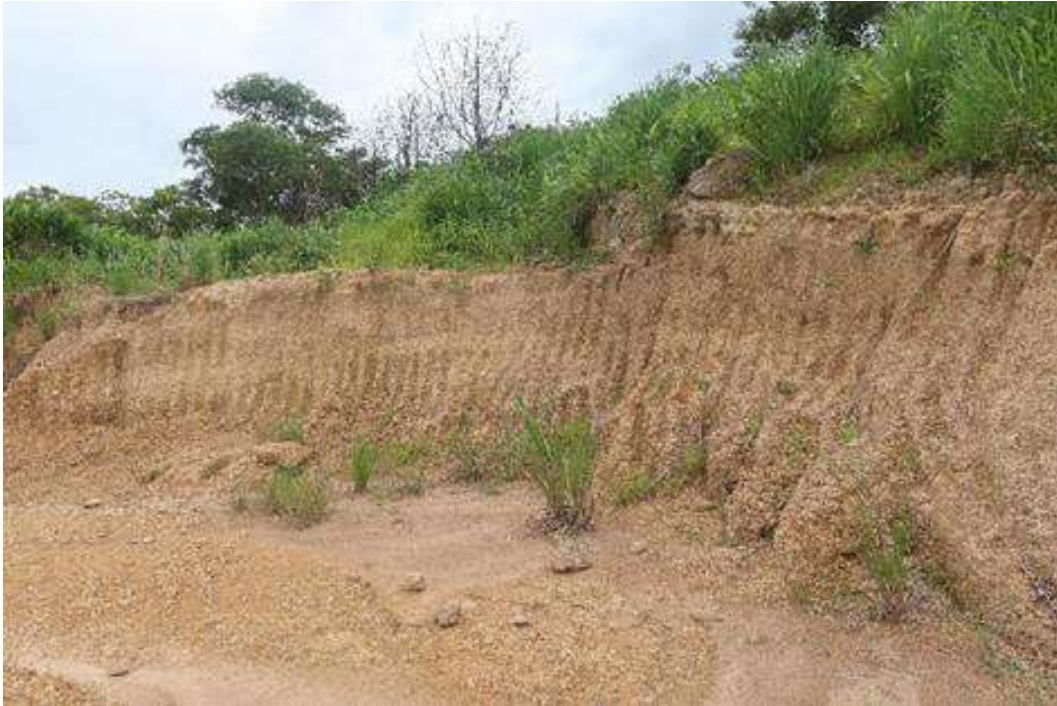
Figure 46 – Photographic record of Reservoir 10 located at PK 132+400.
