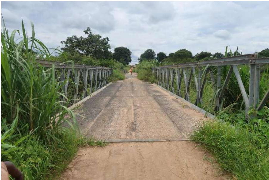
Figure 15 – Photographic record of the bridge located at PK 38+175.
