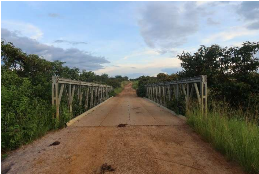
Figure 11 – Photographic record of the bridge located at PK 84+400.
