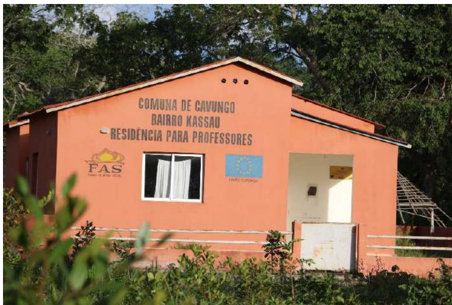
Figure 216 – Photographic record of the residence for teachers located in Comuna de Cavungo – Neighborhood Kassau.
