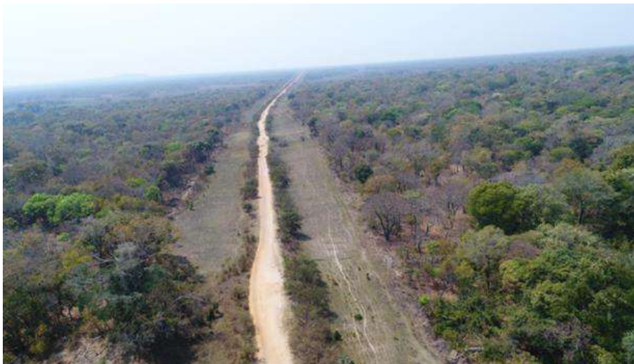
Figure 9 – Photographic record of the end of the road section between Cazombo and Lumbala Caquengue located at PK 70+000 (Source: QG Konstruktion GmbH).
