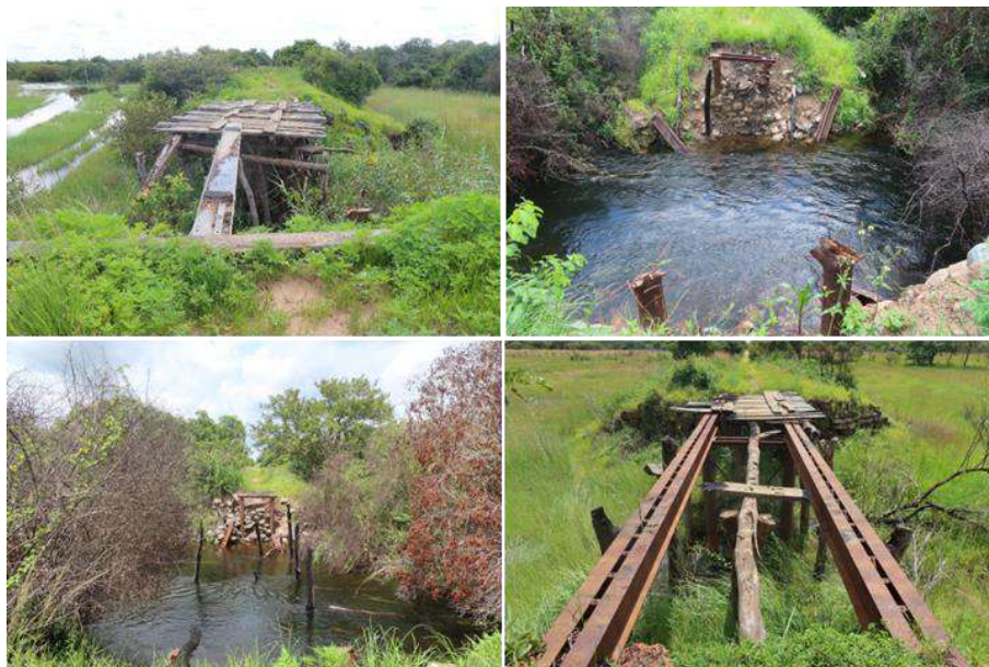
Figure 17 – Photographic record of Box Culverts located at PK 50+590.
