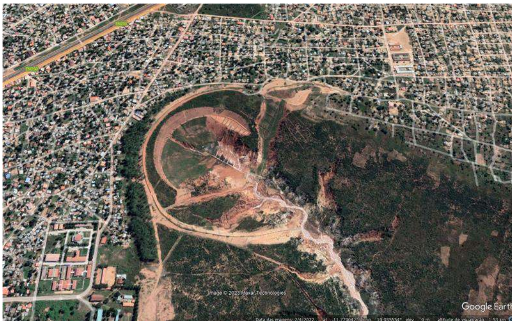
Figure 86 – Existing ravine in the city of Luena (Source: adapted from Google Earth ).
