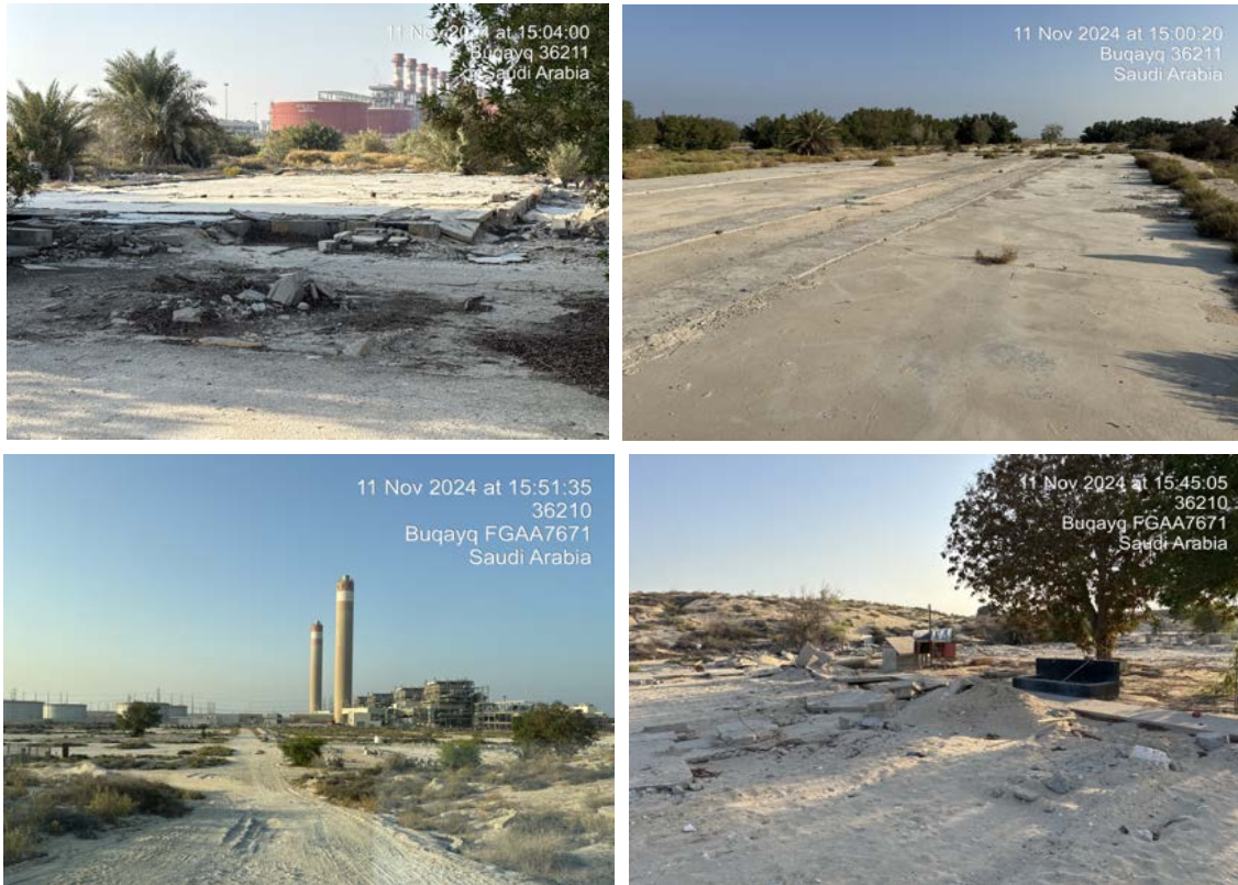
Figure 5-11 Remaining Concrete Foundations, Compacted Road and Demolition Waste at the Project site
