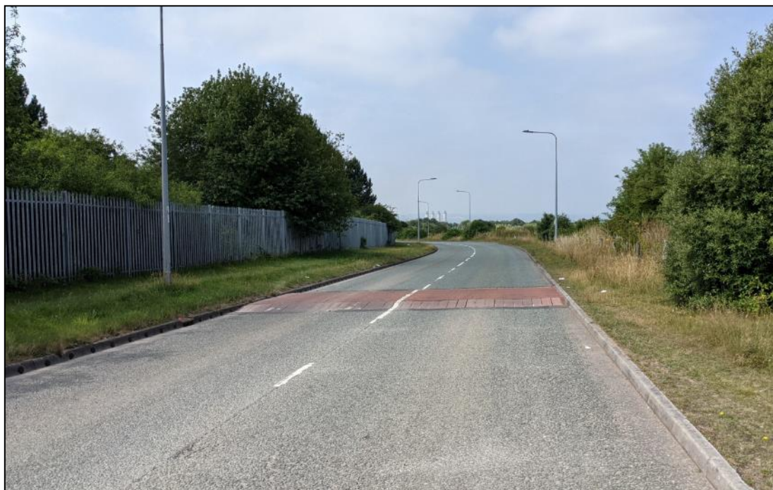
Photograph 13.4: Weighbridge Road (July 2021)
