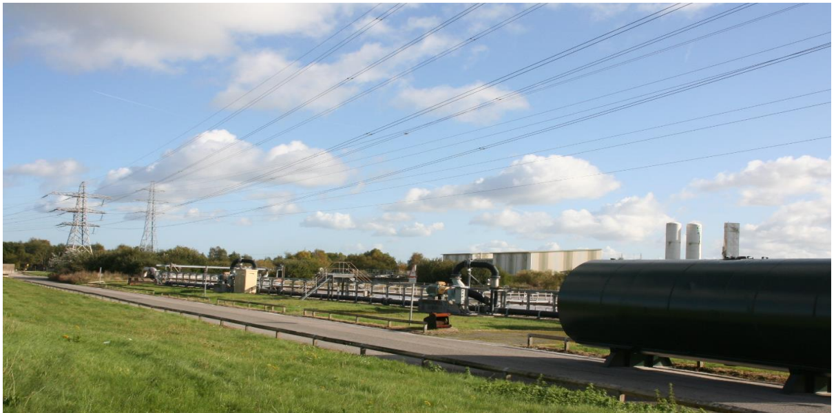
Photograph 2.3 - Utilities infrastructure (October 2021)
