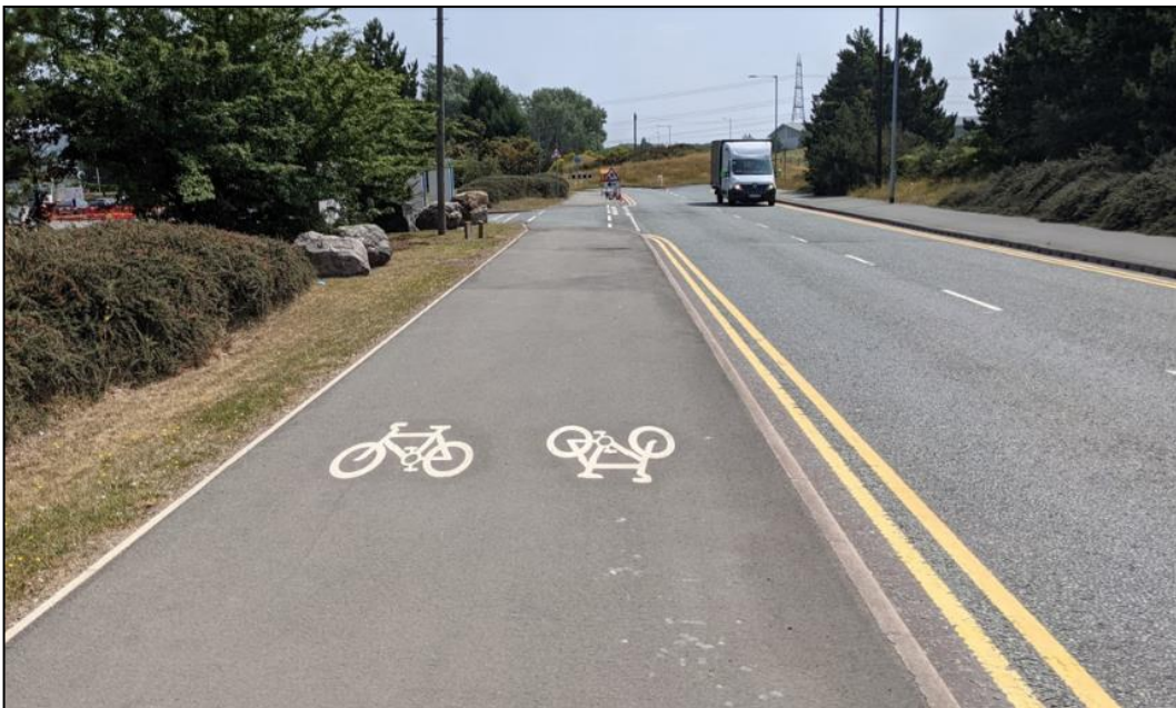
Photograph 13.2: NCN Route 568 Deeside Industrial Estate (July 2021)
