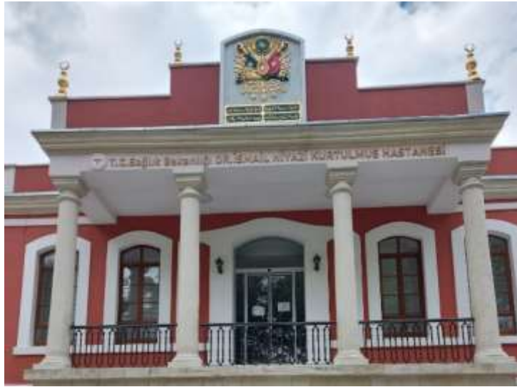
Figure 5-91 Hadımköy Military Hospital
