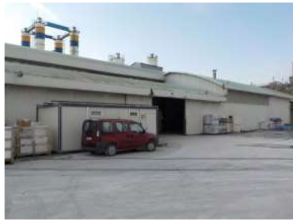
Factory in Ömerli settlement, Arnavutköy
