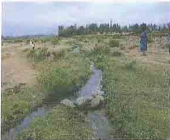
Photo 11: Traditional irrigation canal on right bank of Mersa R. at opposite to station 43+000.
