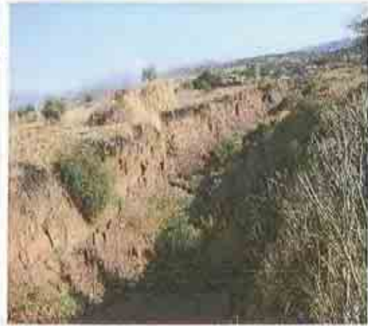
Photo 2: A deep & long gully around km 68 LHS along the road connecting Hara town.
